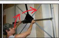
6.Installing the Hanging Rail Place a bin on your shelf and locate how high you want your sliding scale by placing a piece of tape on the upright. Tilt the rail and sliding arm up and push forward until the "half moon" tab disappears into the upright slots.
