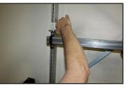
7. Finish Tightening Once you have installed the rail, check for level installation, and use a 7/16" wrench to tighten nuts. Don't overtighten. Repeat as needed.
